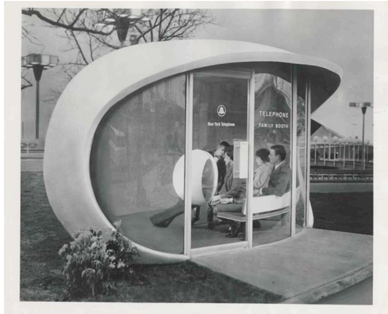
“Telephone Family Booth”
